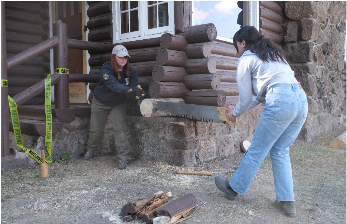
Log Repair at Harriman State Park
