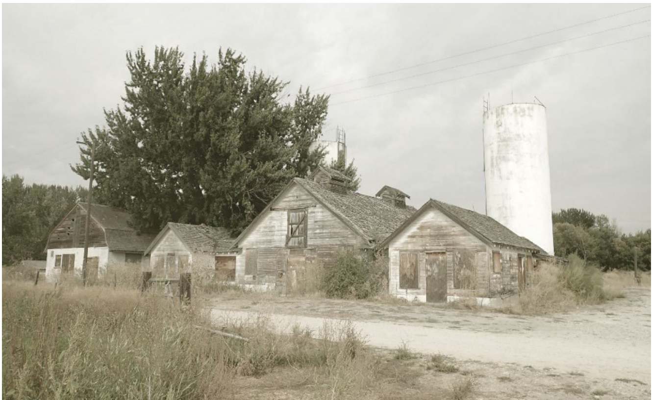
Calf Barn Rehabilitation at Eagle Island State Park
