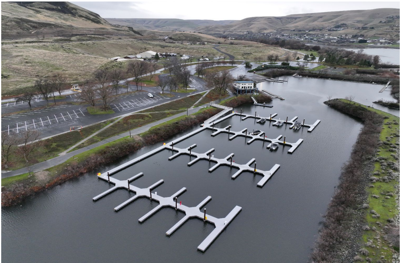
New Marina at Hells Gate State Park
